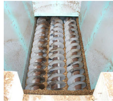
Mounting in discharge screw (wood-fired power plant)
