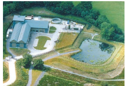
Example of remote pumping station.
