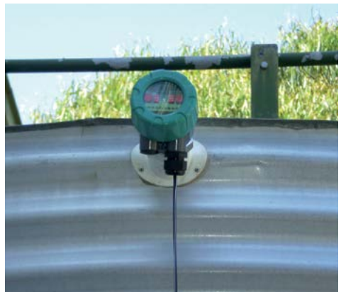
High level switch in plastic pellet silo
